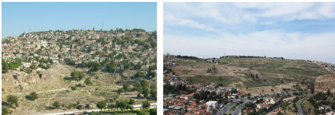
Figure 19. Kadifekale in 2006 and 2011 before and after the implementation of the urban renewal project (IMM, 2018)
